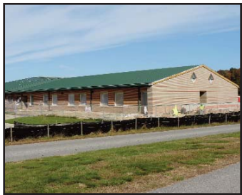
North Georgetown expansion project in early-November.
